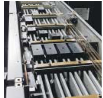
Fully insulated main busbar system.
