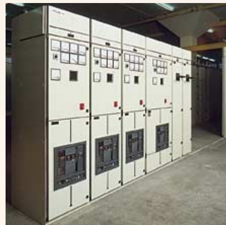
Cubicles with reduced height.
