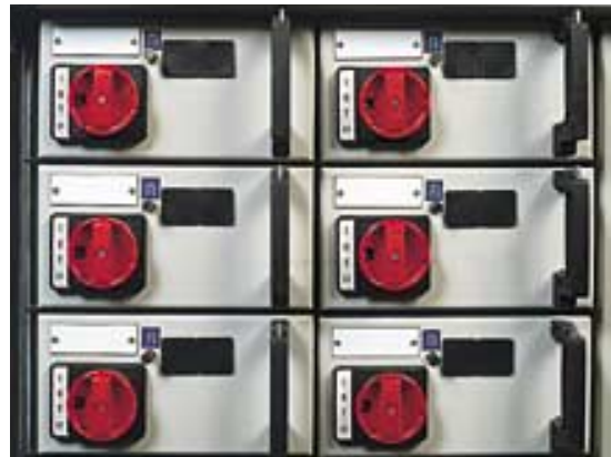
32-drawer system units with fixed front covers.
