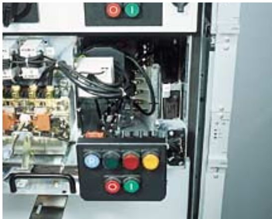
Detail of Capitole 40 cubicle with integrated Clink system. At right (mounted in cable-entry compartment), part of the cassette-mounted Starter Control Units which substitute the auxiliary protection and control devices of each motor starter.
